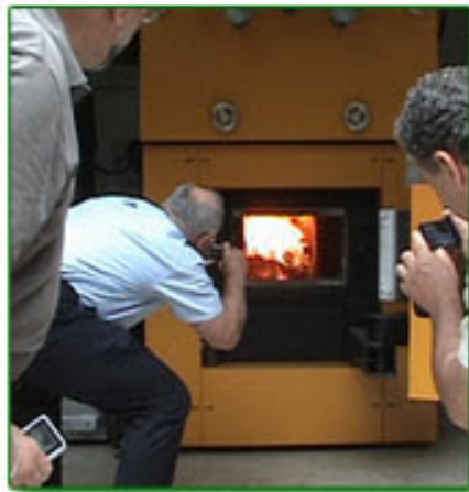
Multi-building renewable energy
